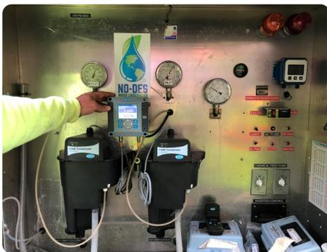
The control panel includes turbidity and chlorine meters to monitor water quality and pressure gages to track filter and pump performance.
