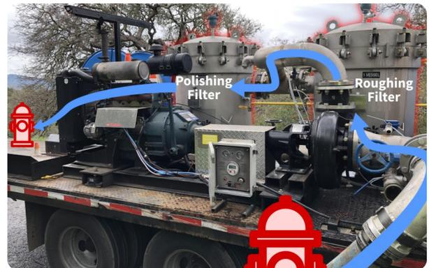
Water taken from one hydrant is sent through two sediment filters in the NO-DES truck and pumped back into the distribution system via a second hydrant. Little to no water is discharged.
